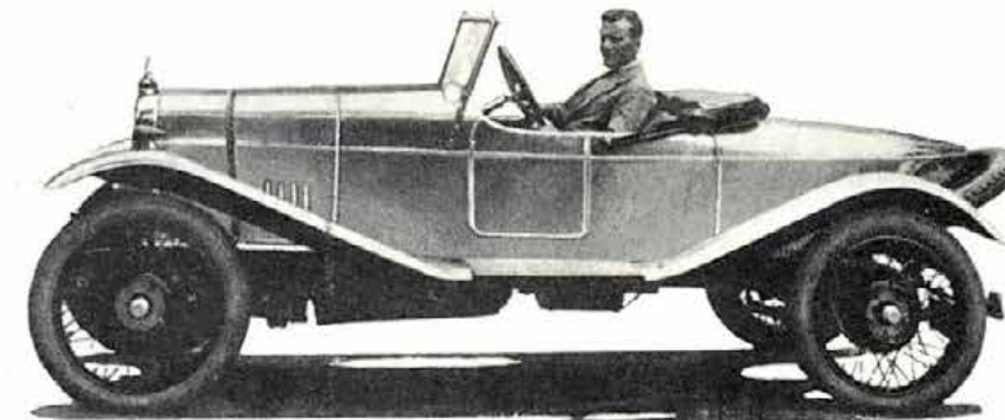
Duck's back: One of Alvis's most famous sports models (above), the 12/50 with aluminium open two-seater body and upturned tail. A racing version won the 1923 200 Miles Race.
